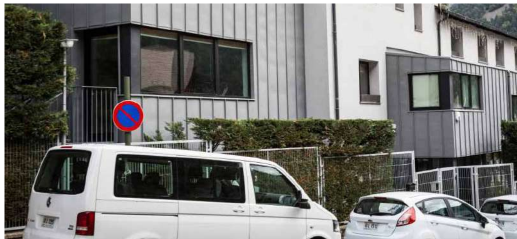
La Gavernera shelter.
