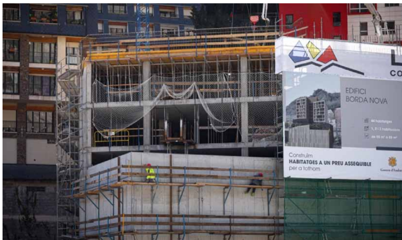
Image of apartments under construction.
