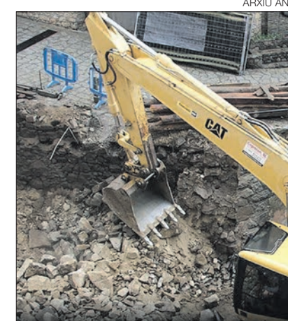
►► A machine works on a construction site.
