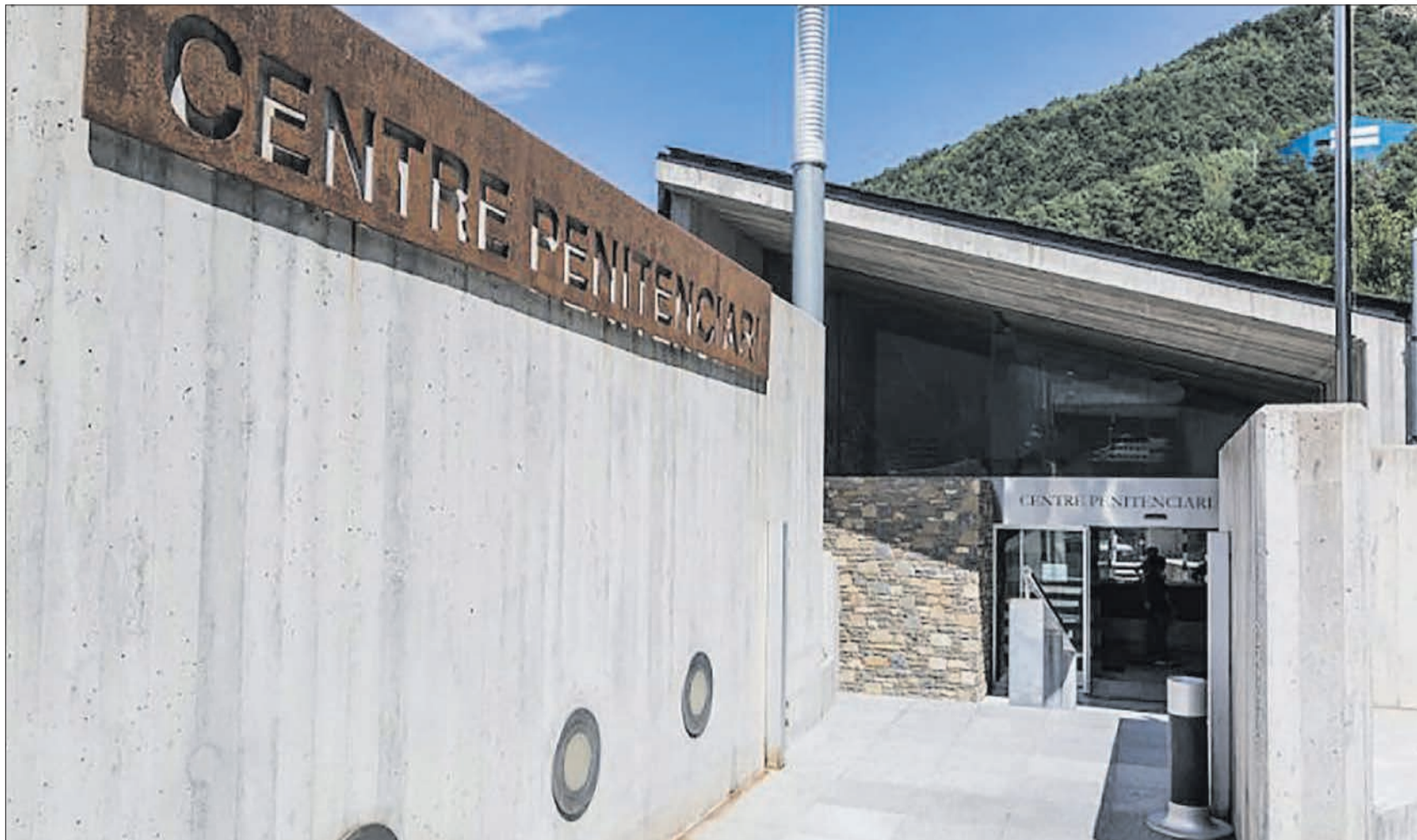
►► Entrance to the Comella Penitentiary Center.
