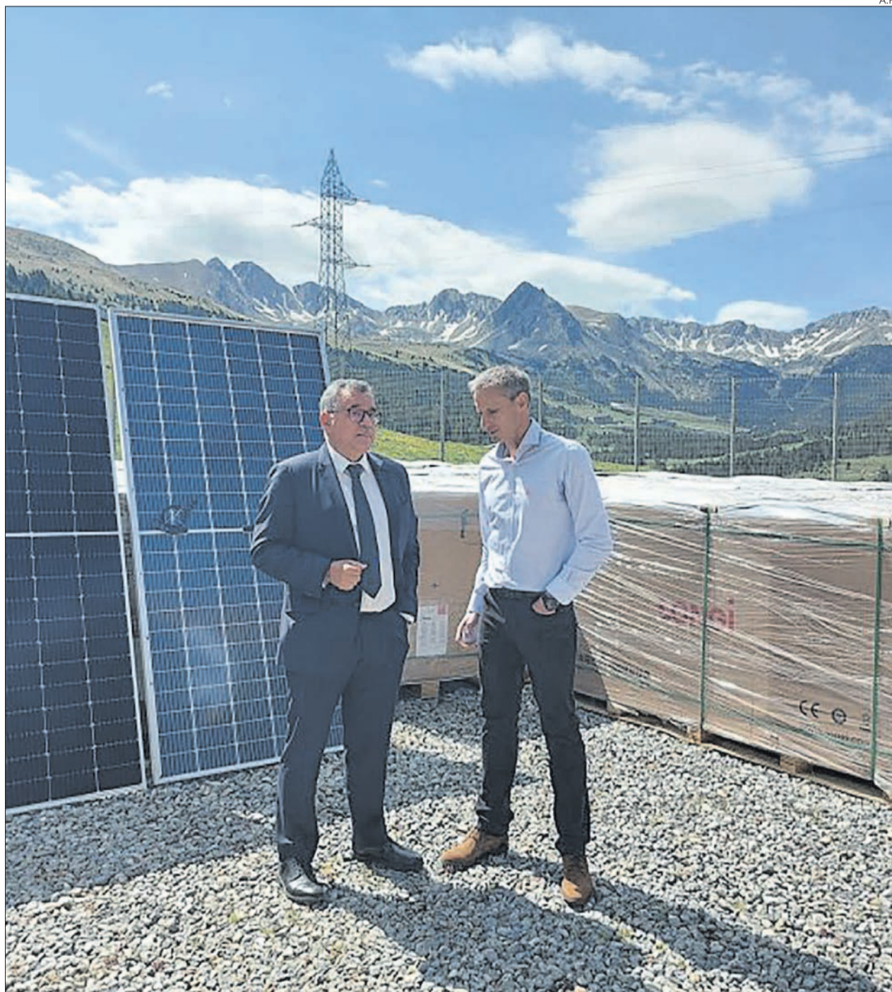
► The director of FEDA, Albert Moles, and the director of Engineering, Marc Calvet, next to the photovoltaic panels of the new solar park.
