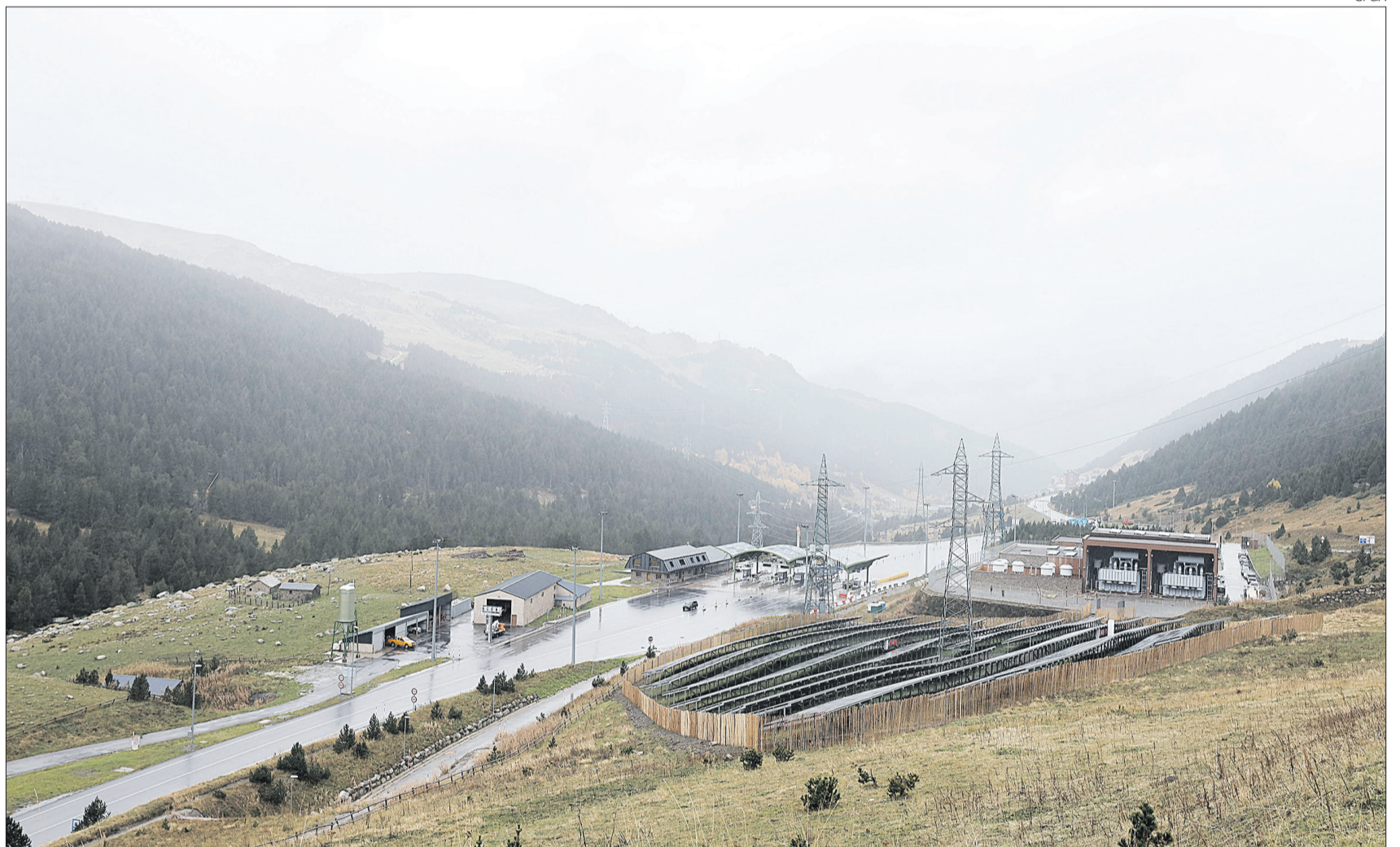
► An archive image of the Grau Roig photovoltaic park.
