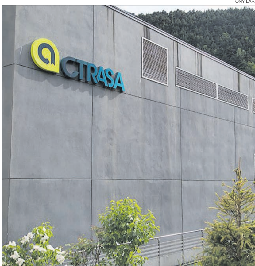
►► The waste incineration plant of the Andorra Waste Treatment Center (Ctrasa) in La Comella.
