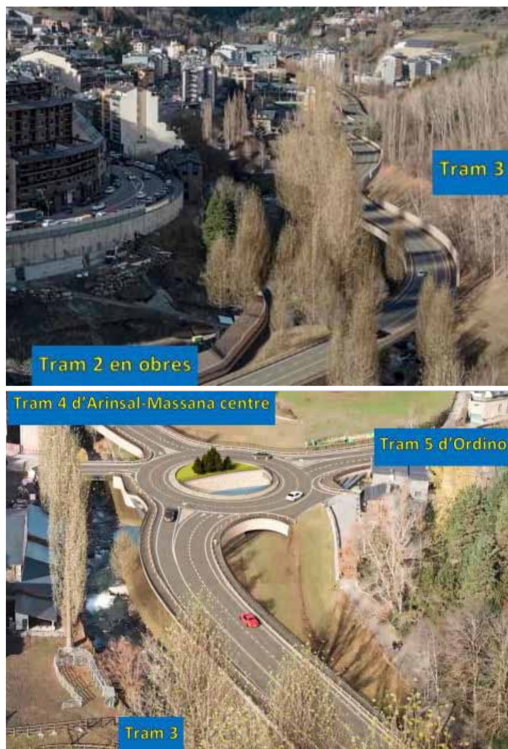
Images of the works project.
