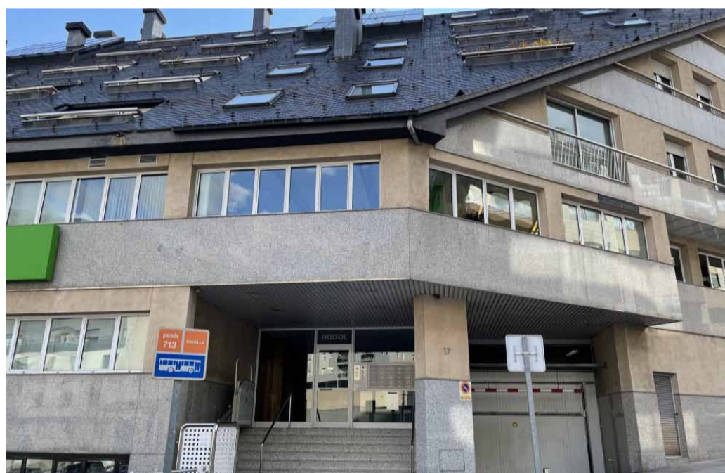
The Ròdol building, located on Josep Viladomat street in Escaldes-Engordany.
